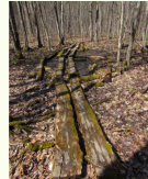
Long plank bridge
